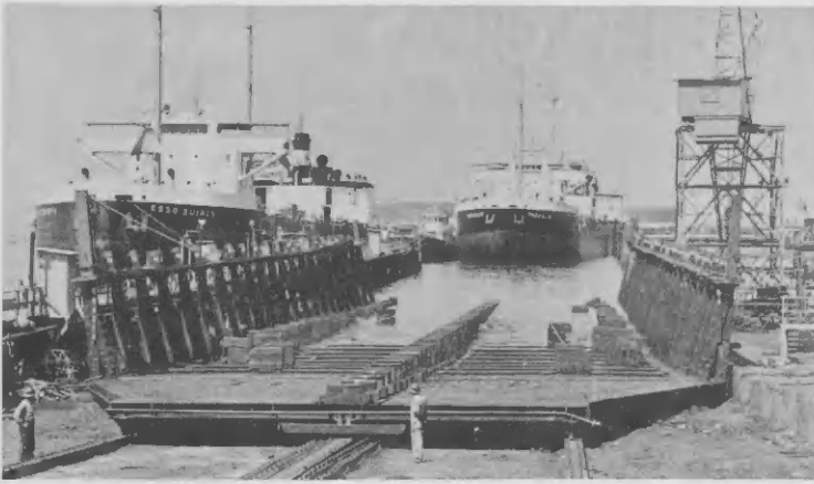
Lago's Drydock where Lake tankers were regularly hauled ashore for repairs or maintenance.
